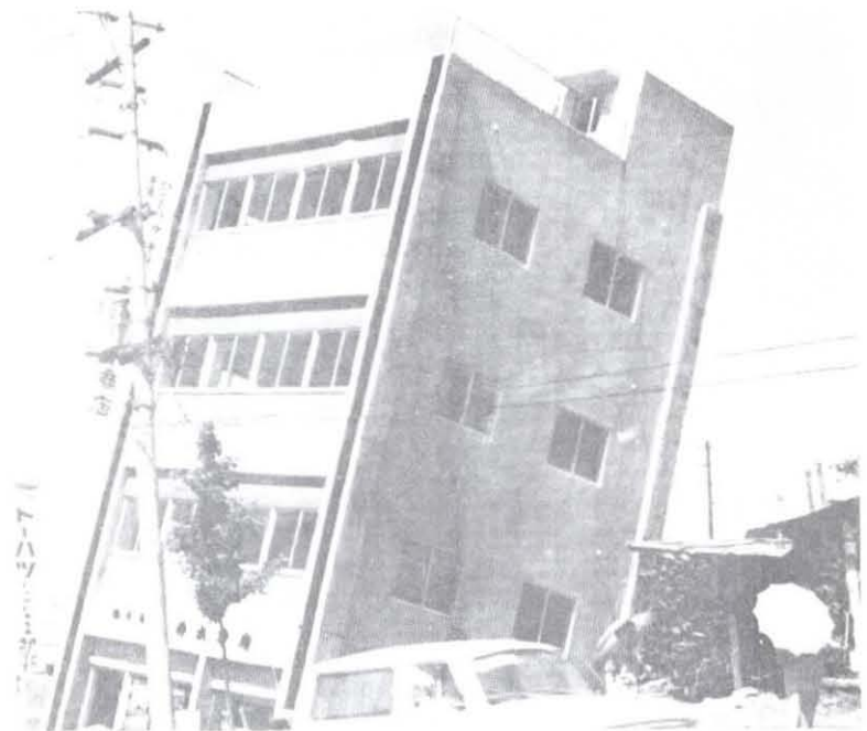
Figure 6 Damage From Ground Instability
